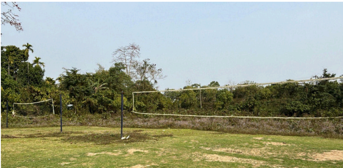
Photo 3: Volleyball Court under construction
